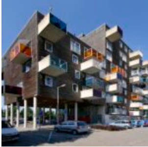
Dwelling for Seniors, Amsterdam, 2016. MVRDV Architects.
