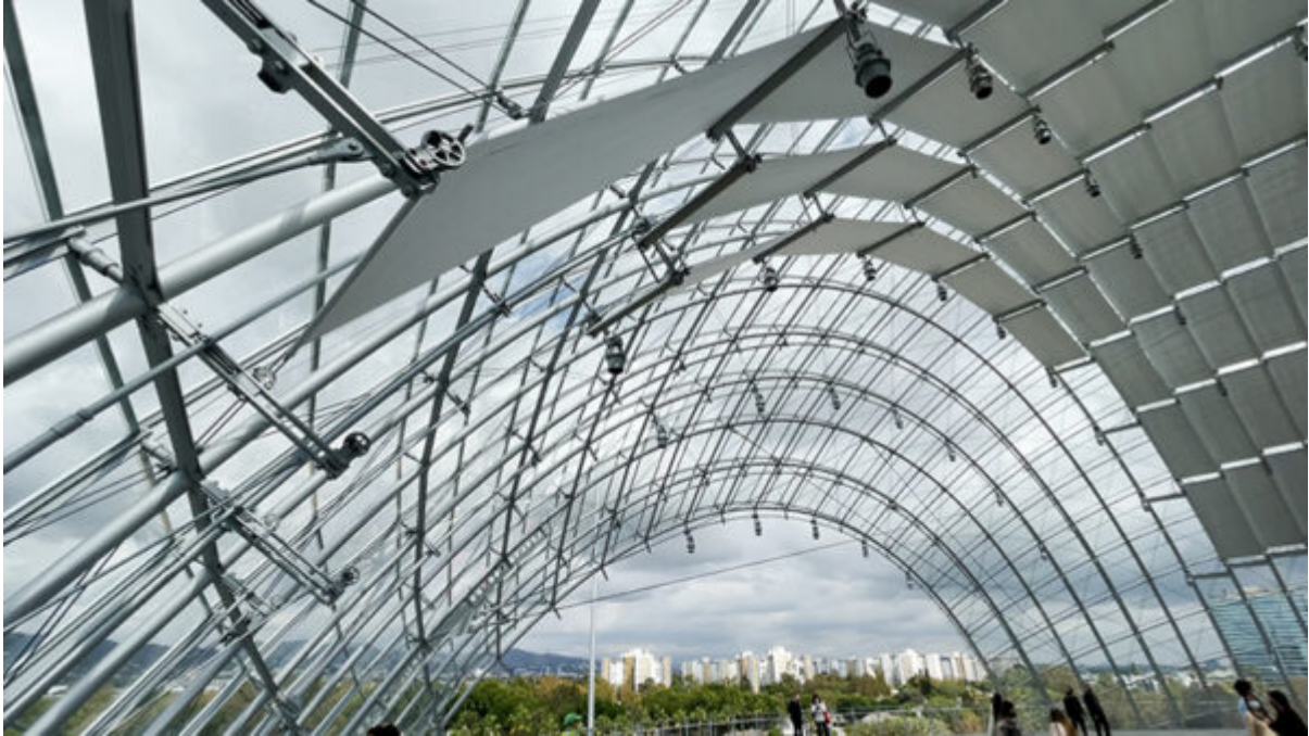
Steel and glass dome over the terrace
