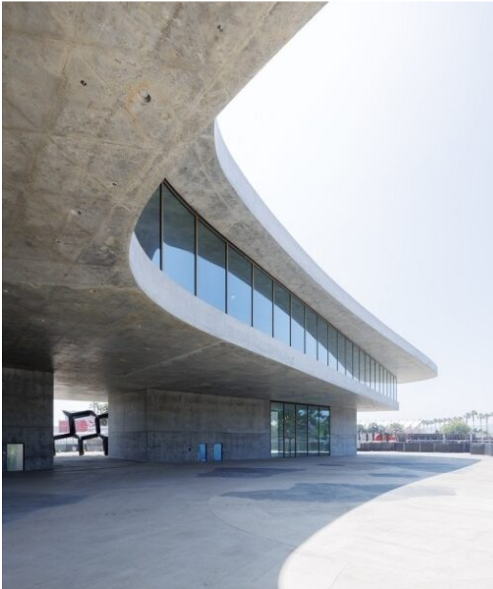
Exterior view of exhibition level of the David Geffen Galleries, photograph © Iwan
