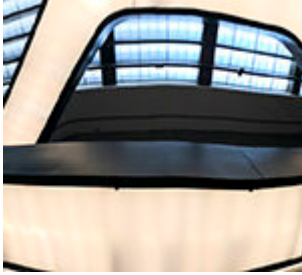
MAXXI – View of ceiling
